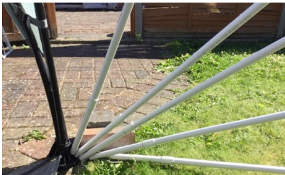
Image 34 · The early stages – using bricks to hold the pipes in place at the canopy hubs
